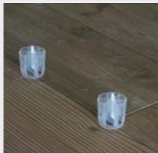
T-shaped leveler installation.
