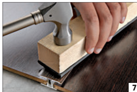
7) With the help of a wooden tapping block, apply pressure evenly over the whole length of the profile using a hammer. If tapping is done correctly, a "click" will be heard when the profile slots into place.
