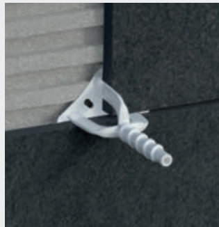
T-shaped leveler installation.
