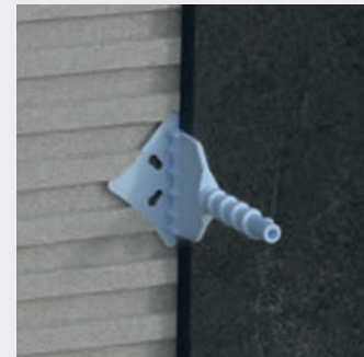
Linear leveler installation.
